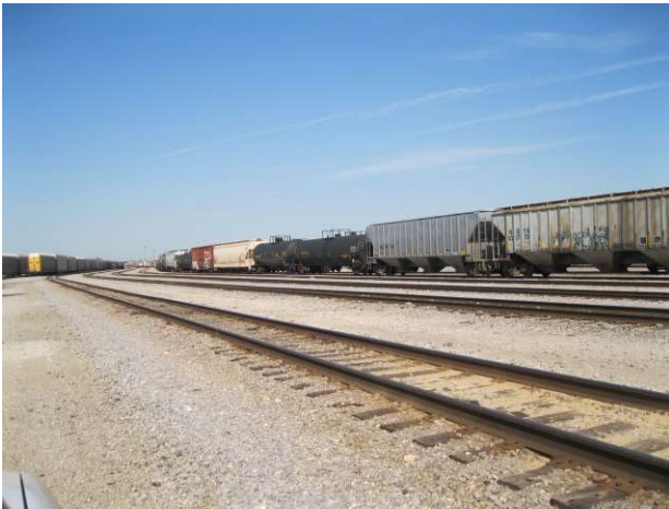
Photos 24 and 25: The Canadian Pacific railroad yard reach contains extensive gravel areas (left photo). The gravel materials improve potential runoff infiltration, provides at least limited filtering of oil, grease, or other materials, and reduces potential runoff volume into Silver Creek. The south parcel of the railroad yard contains office building, parking, and other impervious surfaces. Perhaps the most significant concern (and opportunity for water quality improvement) is the ditch approximately 4,500 LF in length along Franklin Avenue. This non-vegetated ditch contains significant bank erosion, rills, and gullies. During the site visit, vegetated along the ditch was being herbicided (we are uncertain if rock improvement is being proposed along the ditch.) Sediment deposits in the channel bottom are extensive. This ditch is periodically dredged to remove sediment deposits.
