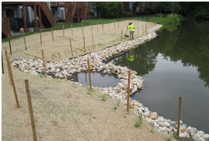
Photo 110: Storm sewer inlets into ponds or detention basins can be modified by constructing sediment forebays (typically the larger the better). Sediment forebays can contain runoff and settle suspended solids before they are carried into the pond area.
