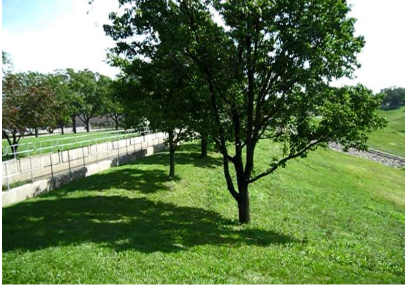
Photo 93: The 50 acre-foot volume Jack B. Williams reservoir in Franklin Park. The concrete-lined Silver Creek channel (at left) completely bypasses the reservoir except during flood flows.
