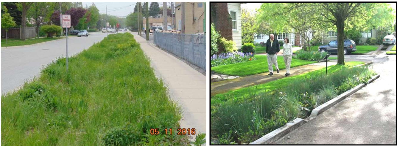
Photos 100 and 101: Urban bioswales can be retrofitted along street rights-of-way to significantly reduce runoff volumes and associated pollutant loading. Signage can help to educate the public.
