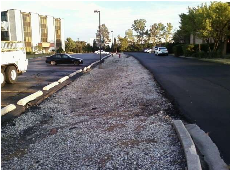
Photo 108: While vegetated areas are preferred, even low-maintenance gravel areas can be used to infiltrate runoff into soils before the pollutants are discharged into the sewer system.
