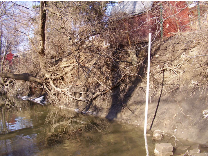
Photos 112 and 113: Before (left) and after (right) example of streambank stabilization on Silver Creek in a residential setting with limited access for construction. BMPs installed by the Village of Melrose Park include re-shaped slopes, vegetation management, rock toe, rock points, boulder energy dissipators (riffles (not pictures), wetland enhancement, and other measures.
