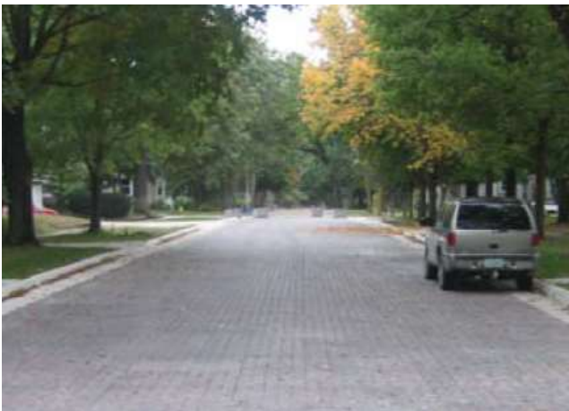
Photo 119: Green streets installed with permeable pavers can reduce runoff volumes by 50% or higher during large rainfall events. Pavers may reduce the need for road salt applications since less ponding will occur. (Source: CDF, Inc. Charles City, Iowa public brochure.)
