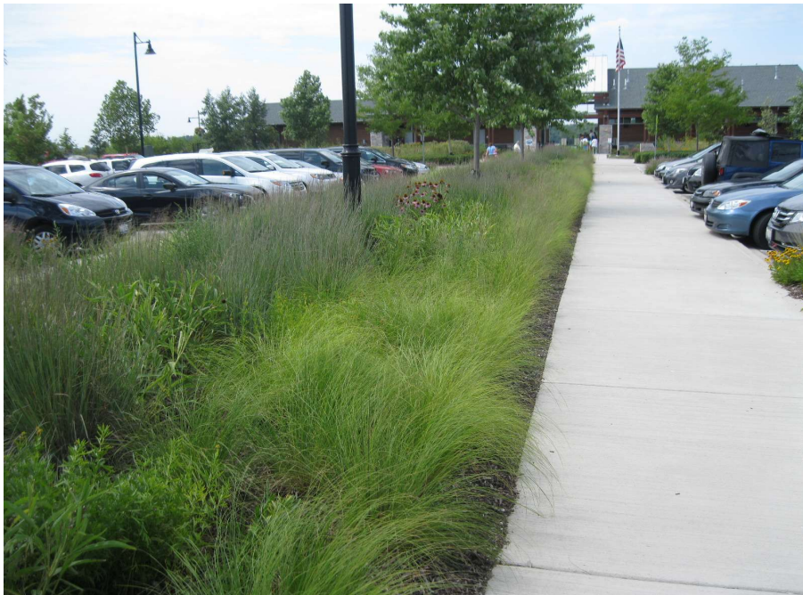
Photo 106: Installation of a linear bioswale with native plants in a setting with expansive parking lots.
