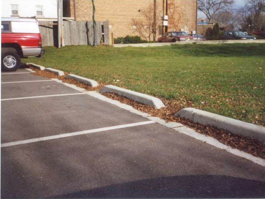
Photo 107: Curb cuts can direct runoff into adjacent vegetative grass filtration areas, rather than collecting 100% of the runoff into the storm sewer system. Treating runoff at the source includes directing it to infiltration areas to the extent practicable. Once runoff enters the storm drain system, all pollutants are then efficiently conveyed into Silver Creek.
