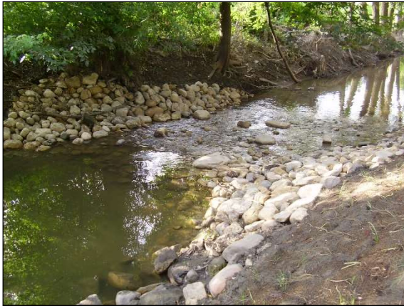
Photos 62 and 63: Dissolved oxygen levels can be improved using instream rock riffle habitat structures to re-aerate the water column. Right Photo: Project Sign for one of the Streambank Stabilization Project Phases informs the public about the Illinois EPA Section 319 Grant Program and the resulting water quality improvement.
