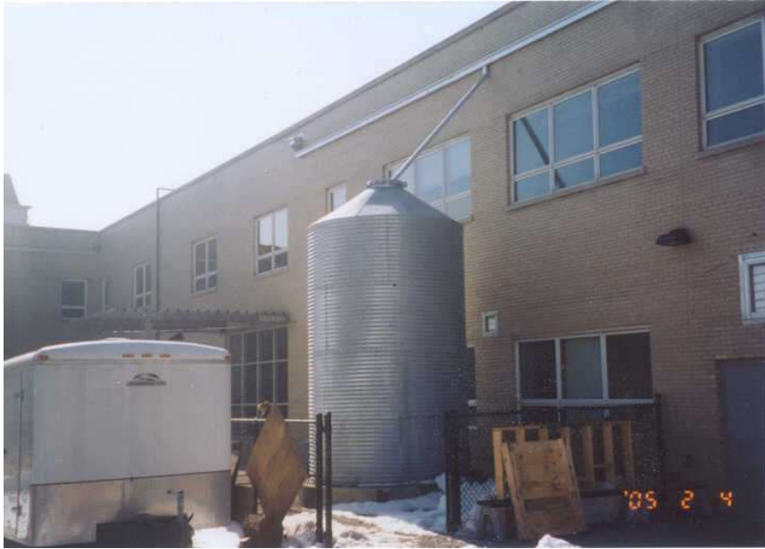
Photo 105: Office building equipped with a large cistern to collect rooftop runoff. Cisterns can be fitted with hoses, or integrated with landscape sprinklers to water the property's landscaping instead of using drinking water. If implemented extensively, cisterns can reduce runoff, pollutant loading, and nuisance flooding in developed areas.
