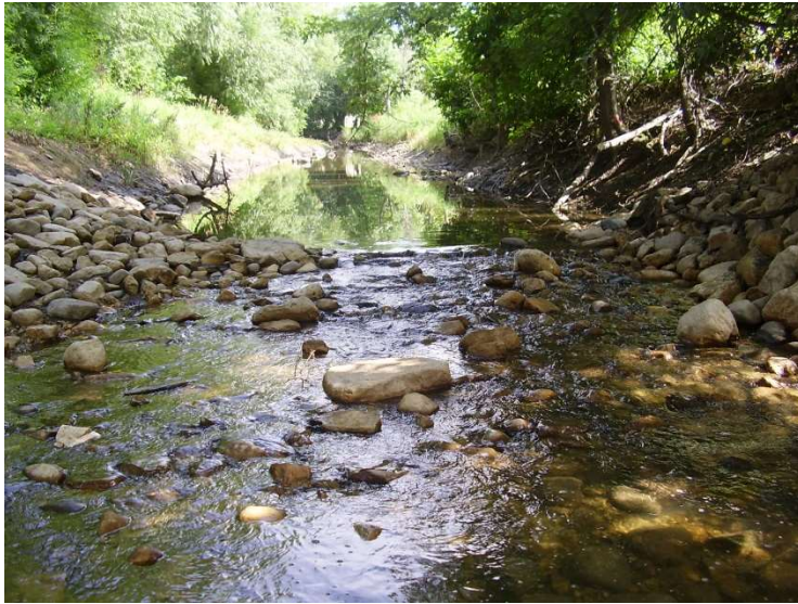
Photo 116: Riffle structures can be installed on Silver Creek to re-oxygenate the water column. This riffle structure on Silver Creek is located approximately 0.5 miles upstream of 5 th Avenue. Riffles also dissipate flow energy, and provide increased habitat diversity.
